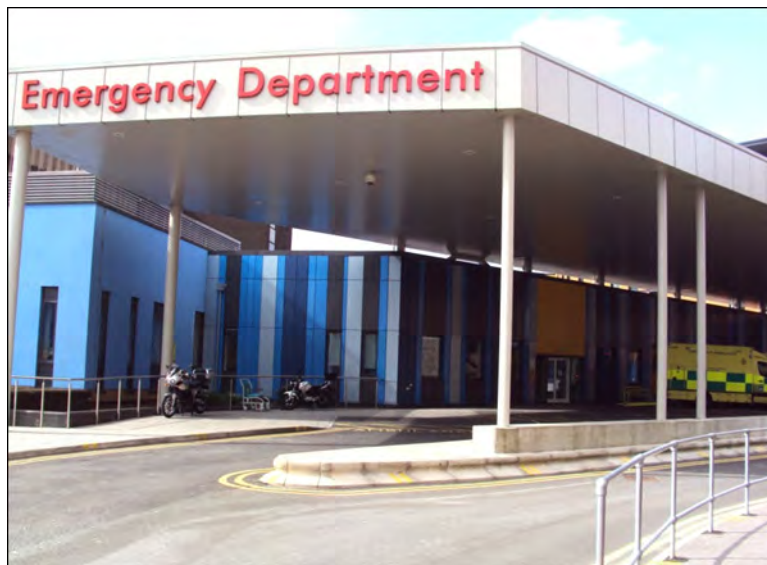
Left: Covered entrance and ambulance bay Salford Royal NHS Foundation Trust Source: Nicholas Cartwright
