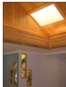
Natural lighting has been enhanced with the insertion of new Velux windows
