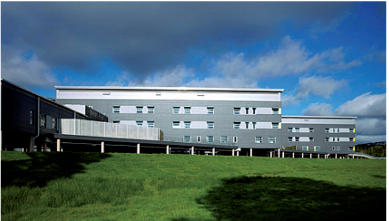
Further view showing elevated building ©Philip Handforth Professional Photos
