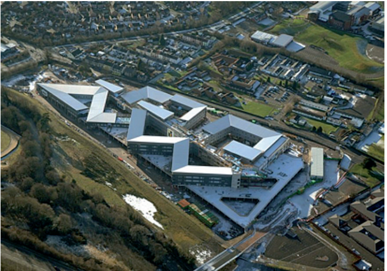
Aerial view of Ysbyty Ystrad Fawr. ©Bam Construction Limited
