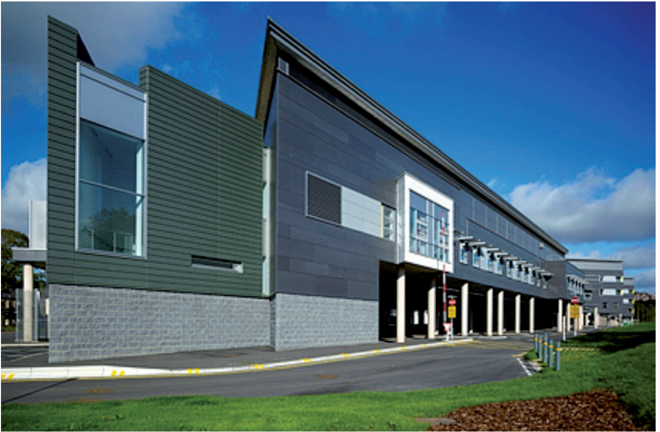
View showing the car park below the elevated building. ©Philip Handforth Professional Photos
