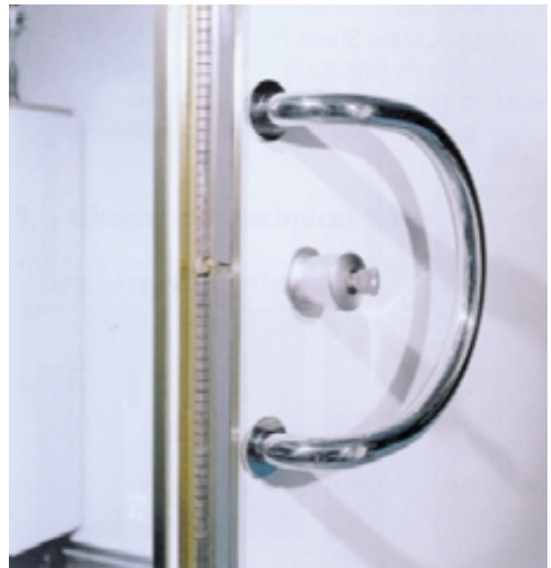
Figure 13.4 Engineering for the integration of a radiofrequency shielded door. Image supplied by lomedco Ltd.
